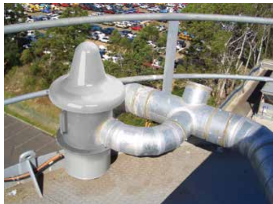
VHS Pressure Relief Valve releasing excess pressure
