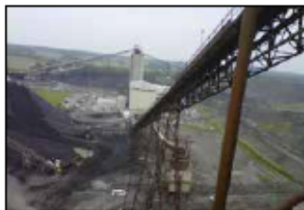
Coal Power Plants A popular sensor for measuring coal and fly ash silos at power plants.
