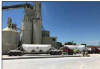
Cement & Concrete Measuring limestone, aggregates, clinker, and finished cement.
