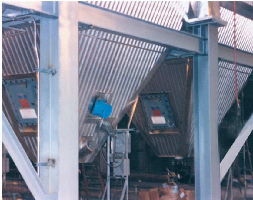
Model V-85 Electromagnetic Vibrator is maintaining flow of dust particulates from the collecting hopper of an electrostatic precipitator.
